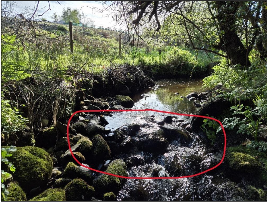
Figure 1-6 - Natural rock to be sealed with small sandbags upon the completion of Dam 2 located downstream of Carrowrevagh Bridge.
