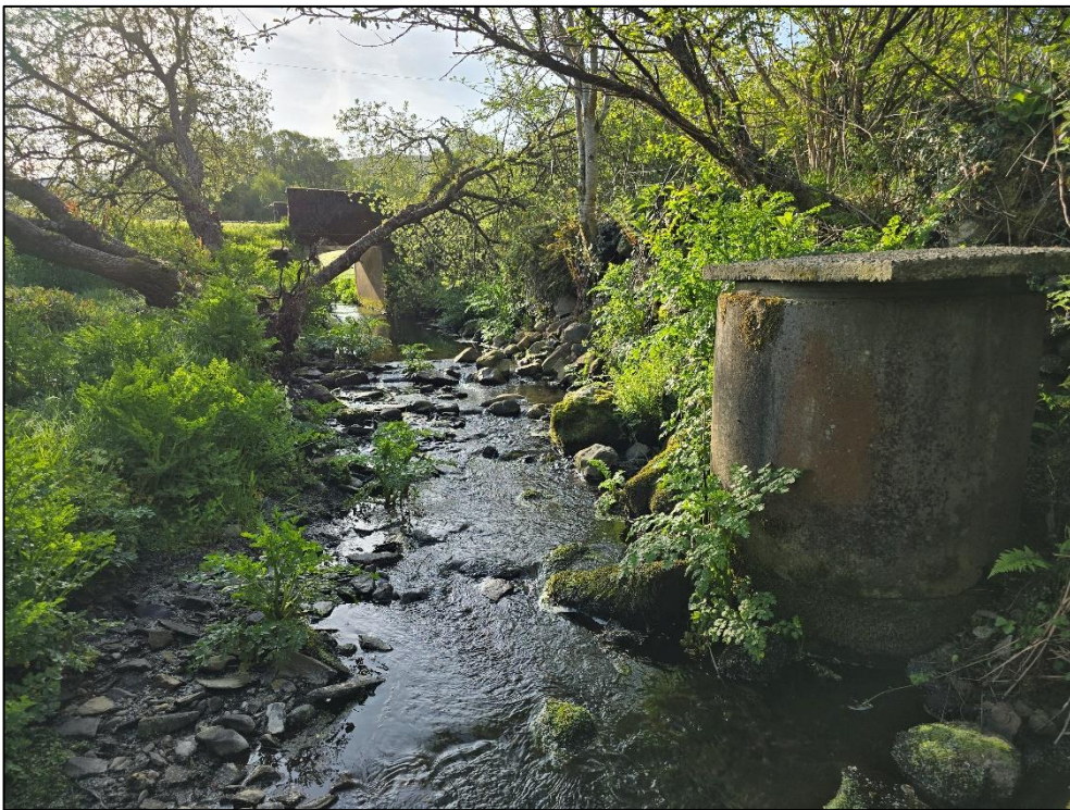
Plate 4-2 – Upstream of Carrowrevagh Bridge facing upstream.
