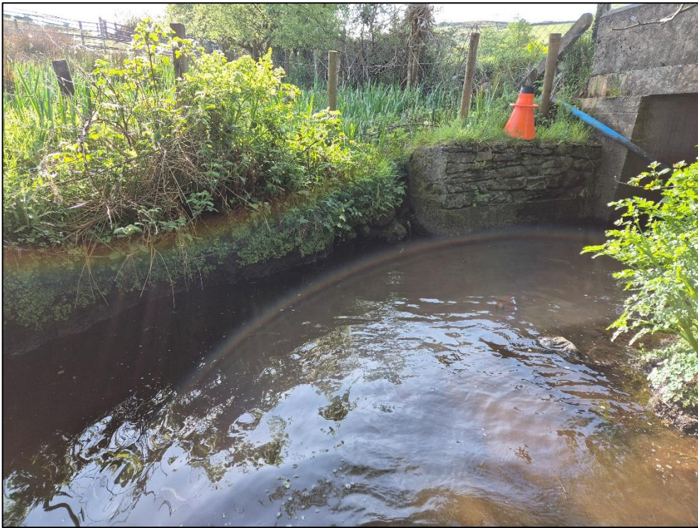
Plate 4-1 – Downstream face of Carrowrevagh Bridge showing concrete section of bridge.
