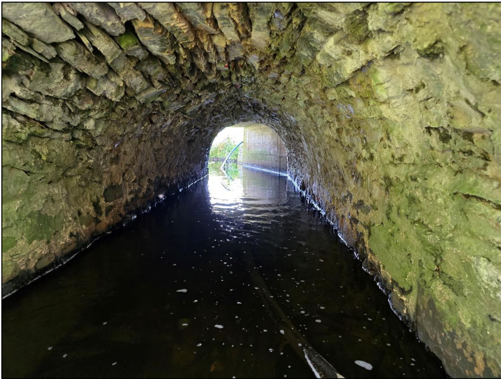
Plate 4-3 - Masonry section of Carrowrevagh Bridge with mass concrete section visible in the background.
